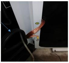
4. Inside the machine you will see the nuts and bolts securing the canopy lid. Undo all the nuts and bolts including the ones at the top at the exhaust end. There are also two nuts and bolts outside on top of the canopy near the lifting hook stickers to undo, then remove the canopy lid. The machine should now look like this:
